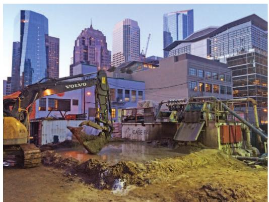
ings, the shafts were drilled to pile tip elevations using a CZM EK-250\* Drill Rig. We used bentonite slurry to help maintain the shaft stability during the drilling operations. Bentonite slurry was very successfully in maintaining the shafts side walls through the varying subsurface conditions. Some of the shafts took multiple days to drill due to the varying hardness of the rock within the Franciscan complex.
